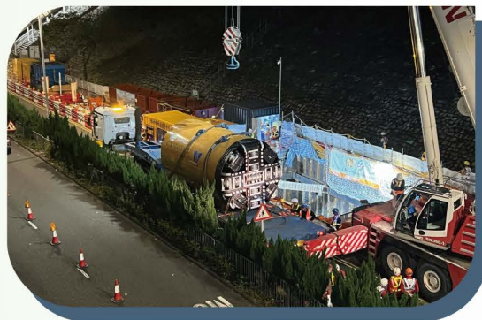
第一段頂管隧道工程展開 First section of pipe jacking tunnel works commenced
