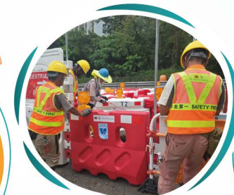
加固水馬及移除檔板 Reinforcement of Water Barriers and Removal of Baffles
