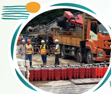
加設擋水版 Installation of Flood Barriers
